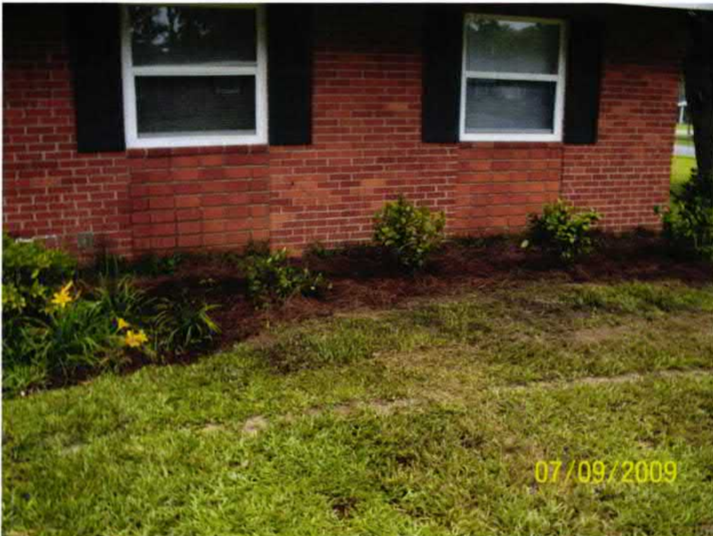
Picture 2: Site after completion of work.
