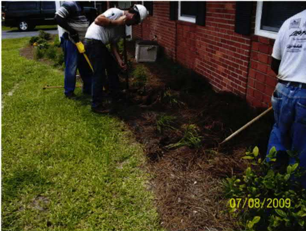
Picture 1: Location of UST 1371Dove prior to removal.
